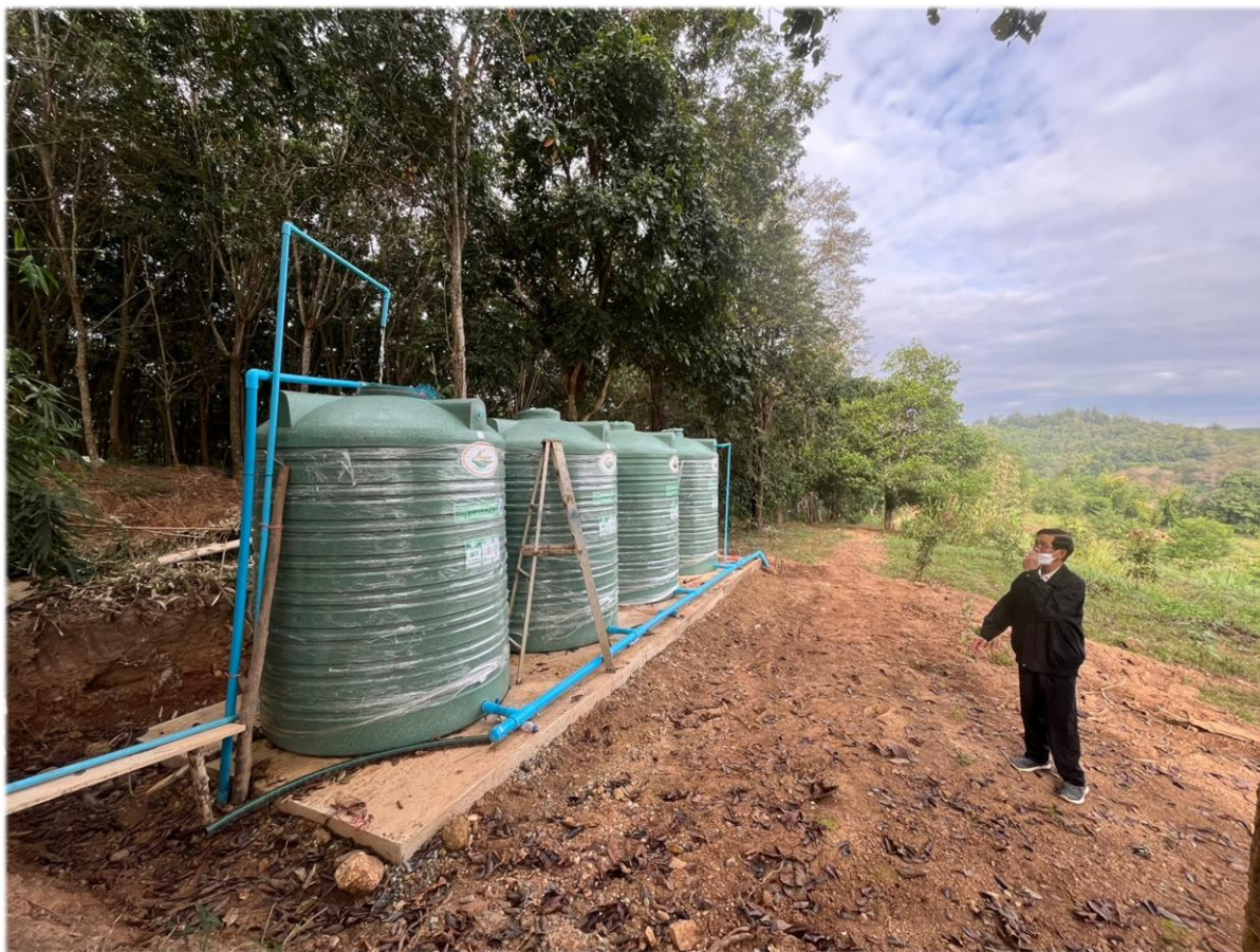
Bua Yai Subdistrict, Na Noi District, Nan Province: Water system for solar irrigation. Source: Authors.
